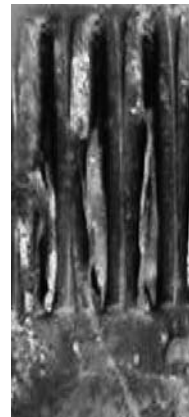
Example 2: PPL separated from base metal due to sulphuric acid attack
